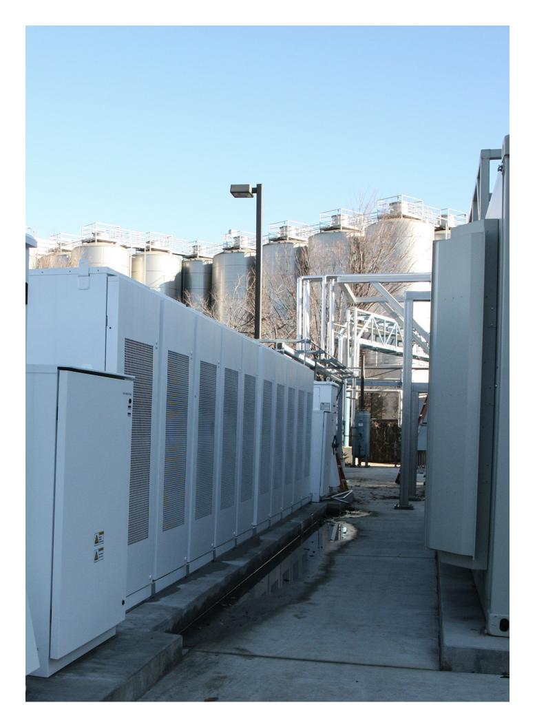
The 1 megawatt-hour of Powerpack batteries holds enough energy to drastically reduce the brewery's demand charges. (Photo credit: Sierra Nevada)
