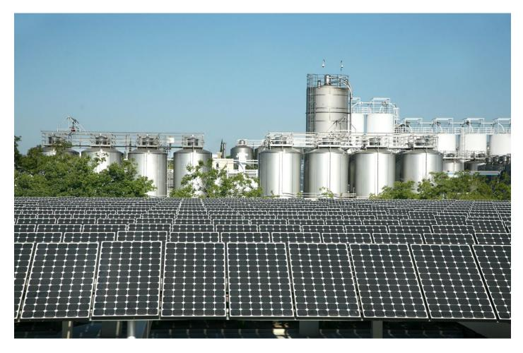
Sierra Nevada's 10,751 solar modules generate 2 megawatts of power and offset 20 percent of the brewery's annual electricity consumption. (Photo credit: Sierra Nevada)
